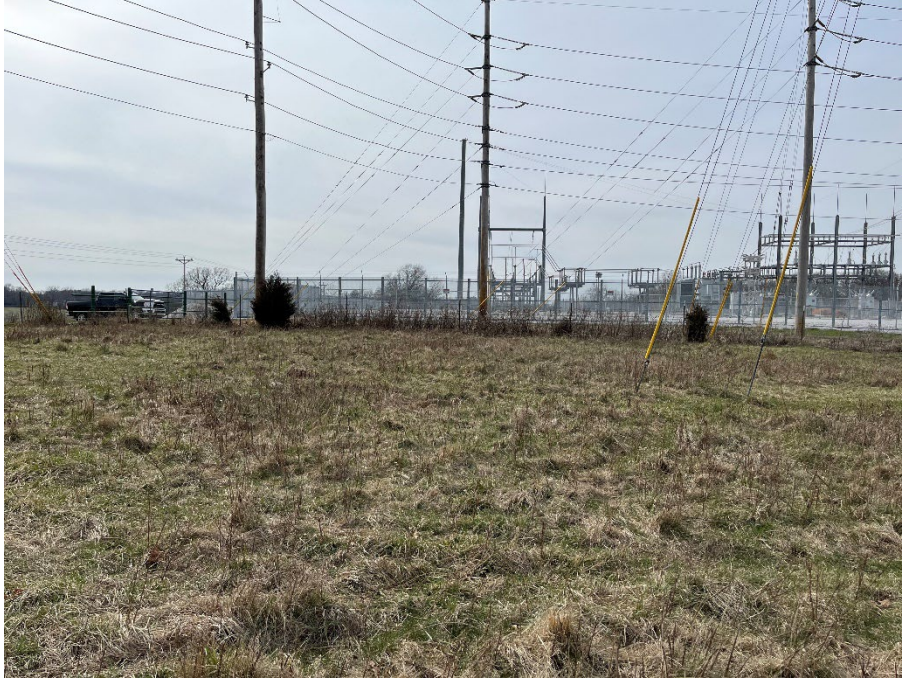
Photo 3: Transmission line and substation in southern half of Project area facing west
